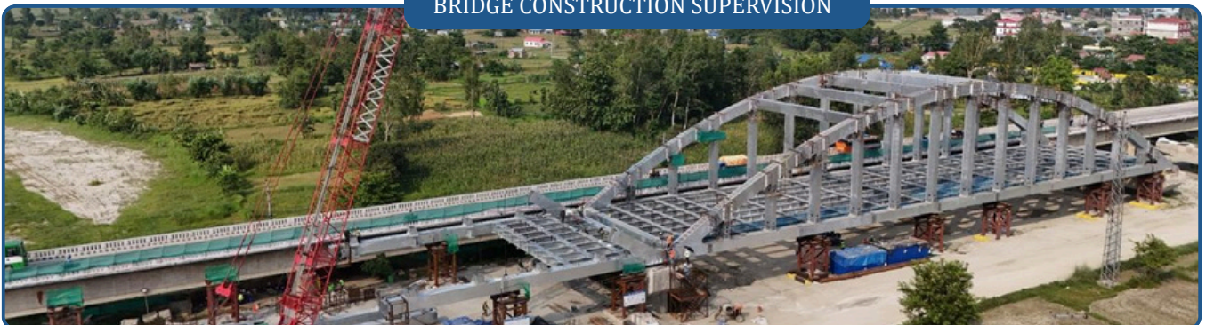
BRIDGE CONSTRUCTION SUPERVISION
