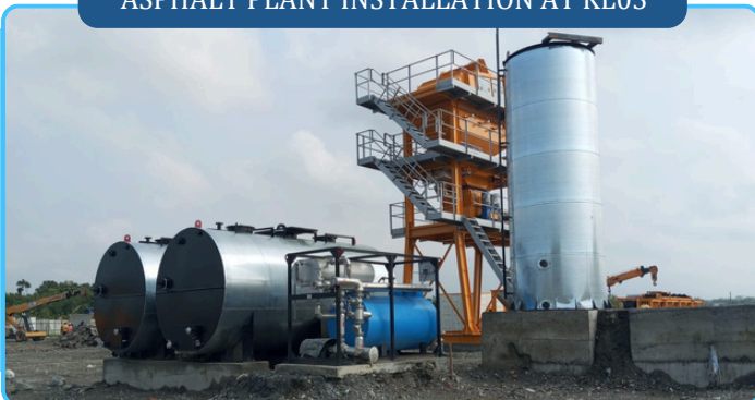
ASPHALT PLANT INSTALLATION AT KL03
